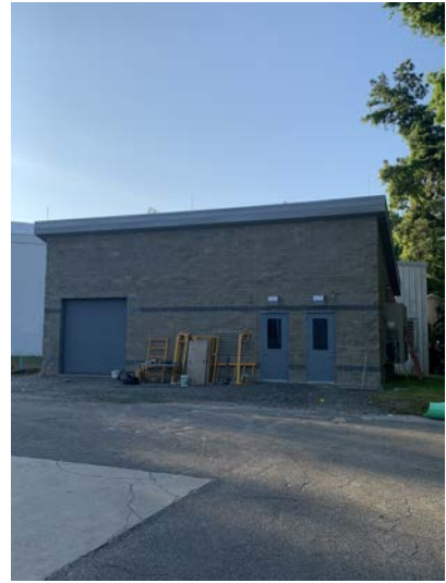
High Service Pump Station
